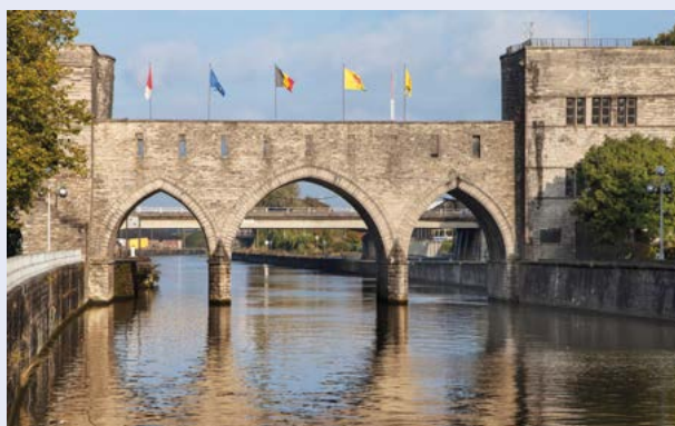
Pont des Trous/Gatenbrug over the Schelde River, Tournai, Belgium.
