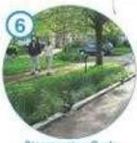
6 Bioretention Curb Extensions
