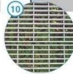
10 Walkable Steel Grating Over Recessed Planters
